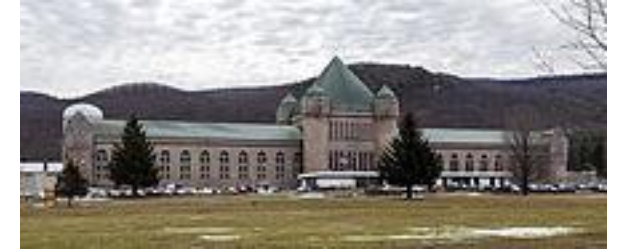
Eastern Correctional Facility in 2015 Source: wikipedia
